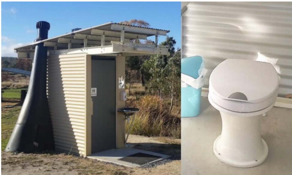
Figure 2-7 Example evaporating toilet for trail top.
