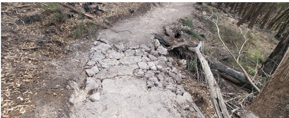
Figure 2-2 typical example of rock armouring
