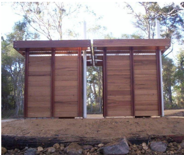
Figure 2-5 Example below of a prefabricated double toilet block structure used extensively through NSW State Forests
